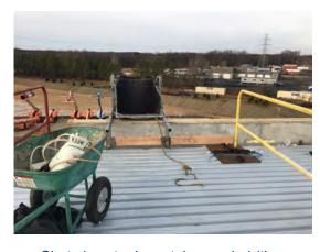
Chute is guarded on both sides to prevent workers from falling when dumping.
