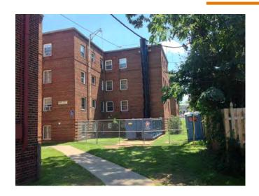
In order to prevent against people standing near the dump area when you're dumping material from the roof into the dumpster, barricade your dumpster and chute area. As seen in the picture the dump area is barricaded by a fence.
