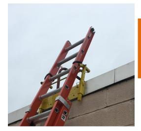
The top of the ladder should be secured either by a ladder securement device (like shown in the picture) or by tying the ladder to the roof using ropes or adjustable tie-downs.
