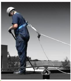
This worker cannot reach the edge and cannot fall, called "Fall Restraint".
